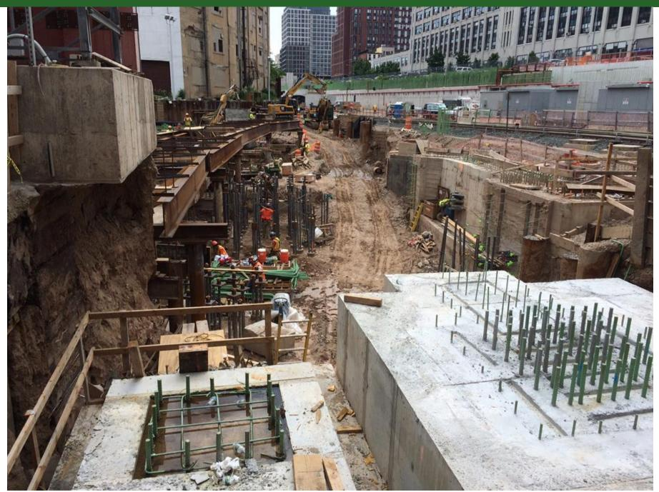
LIRR YARD - Footing and Shear Wall Construction
